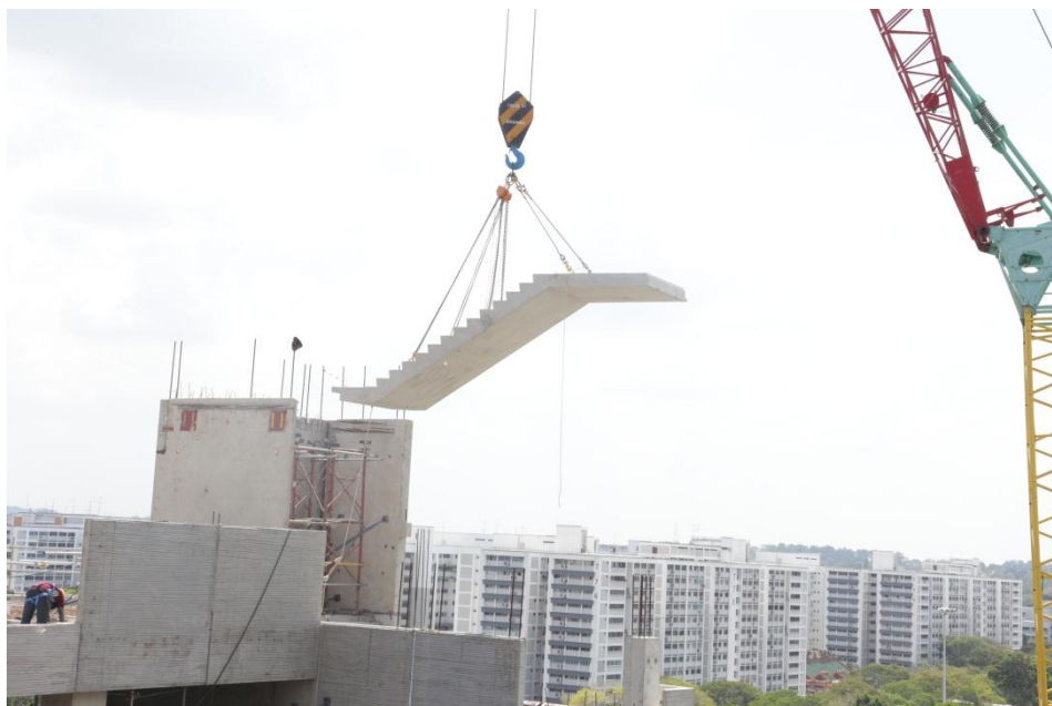
A pre-fab staircase being assembled on site.
