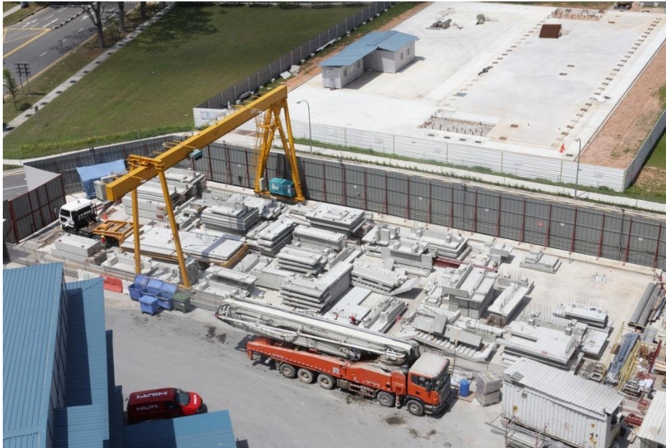
A pre-fab yard onsite helps to facilitate the construction process of YCH through time savings.
